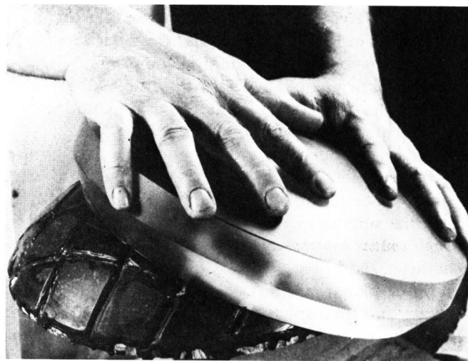
Figure 5.7 Polishing a spherical lens. (Photo courtesy Optical Society of America.)
